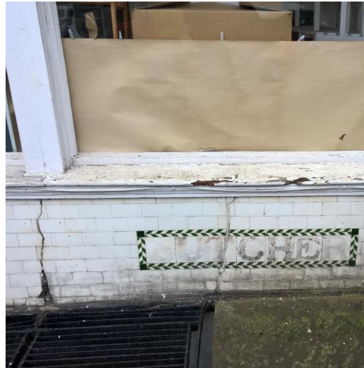
Original tiling / signage to shopfront
