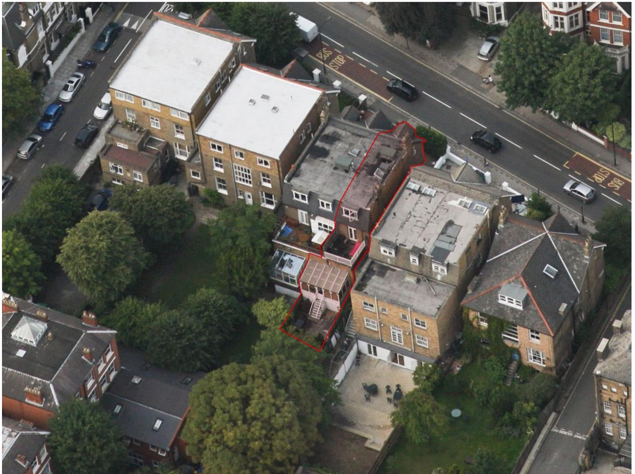
Arial View-Site Subject to Planning
