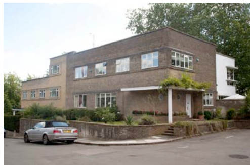
Figures 3-5: Modernist houses Sun House, Frognal Way, No. 66 Frognal & houses in Frognal Close
