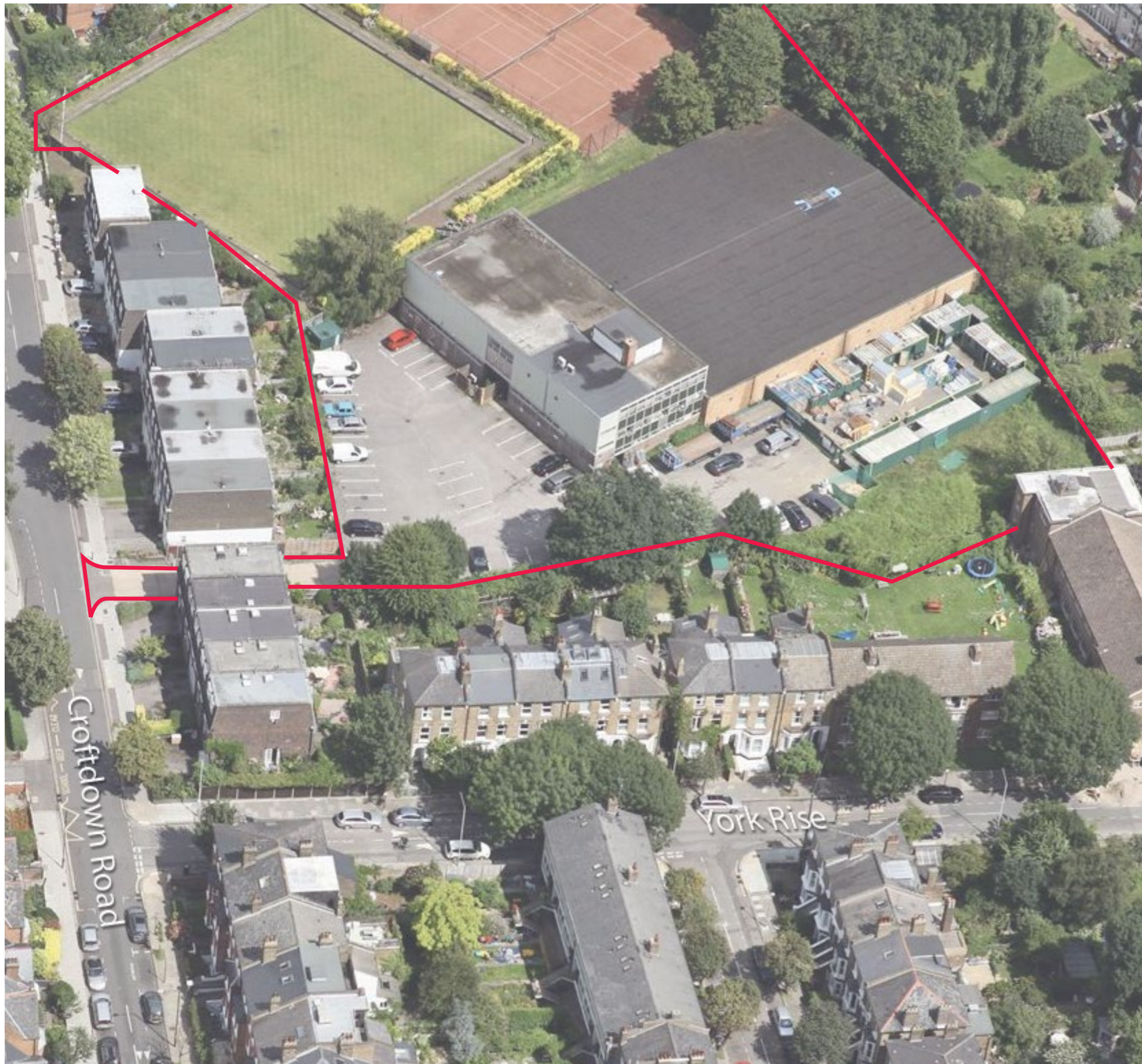
Aerial view from the West
