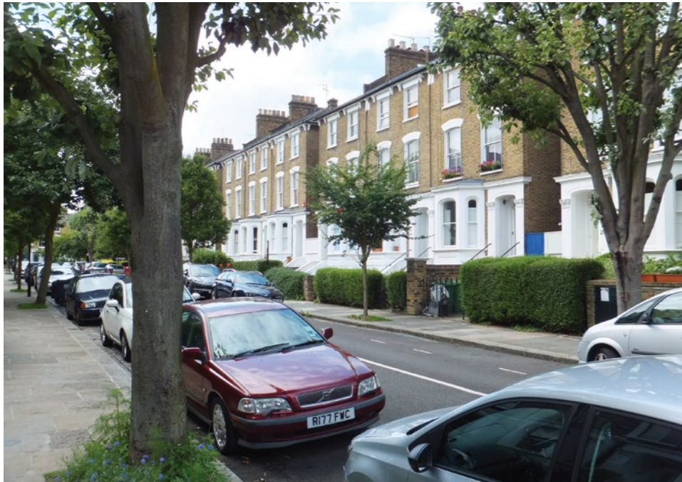
Laurier Road Victorian town houses have ground floor levels highlighted with render and upper levels of London stock brick. Windows are vertical in proportion and often have white painted reveals.
