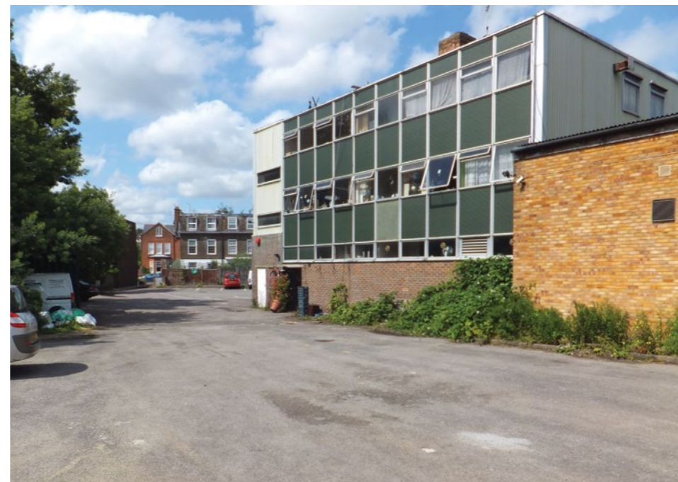
Southern elevation of clubhouse View along the southern façade of the clubhouse towards the main vehicular entrance on Croftdown Road
