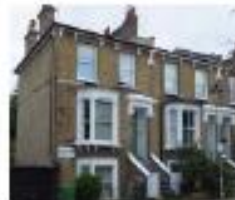
Terraced houses - Woodhouse Road
