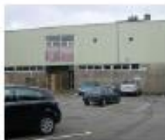
View of current MRC building from entrance
