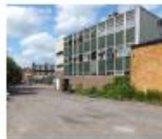
View of current MRC building
