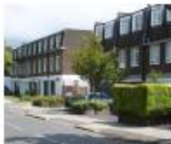
Site entrance - Craftdown Road
