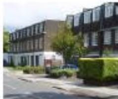
Site entrance - Croftdown Road
