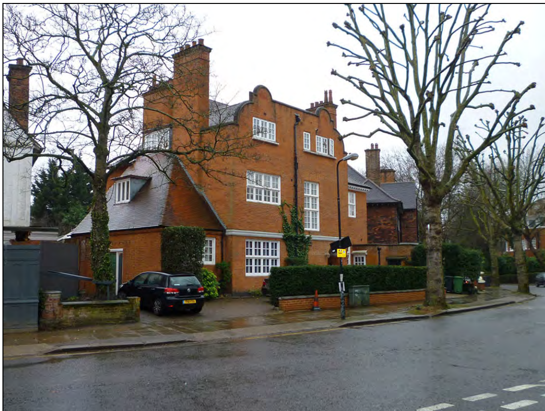
Fig. 2 – Front elevation viewed from the north east, with No. 57 to the right of the image
