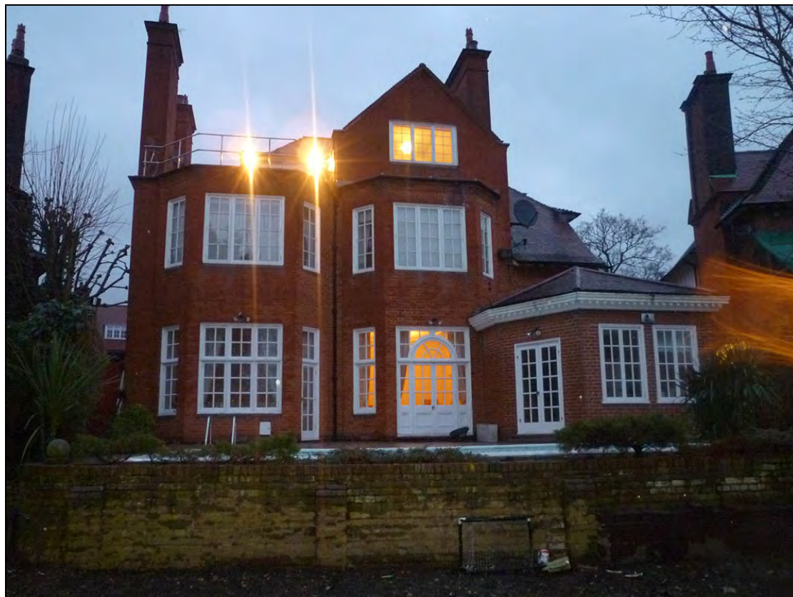
Fig. 4 – Rear elevation looking south west, with No. 53 to the right
