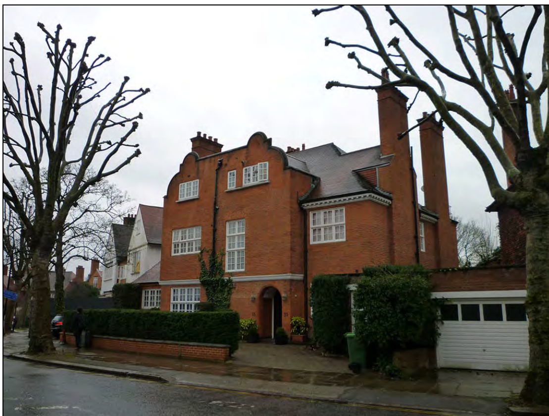
Fig. 3 – Front elevation looking from the north west, with No. 53 in the background
