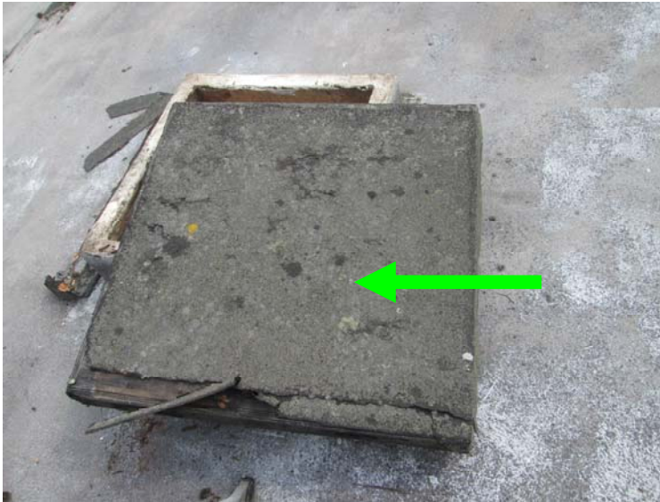
Sample 01 – Roofing felt to loft hatch - no asbestos detected.
