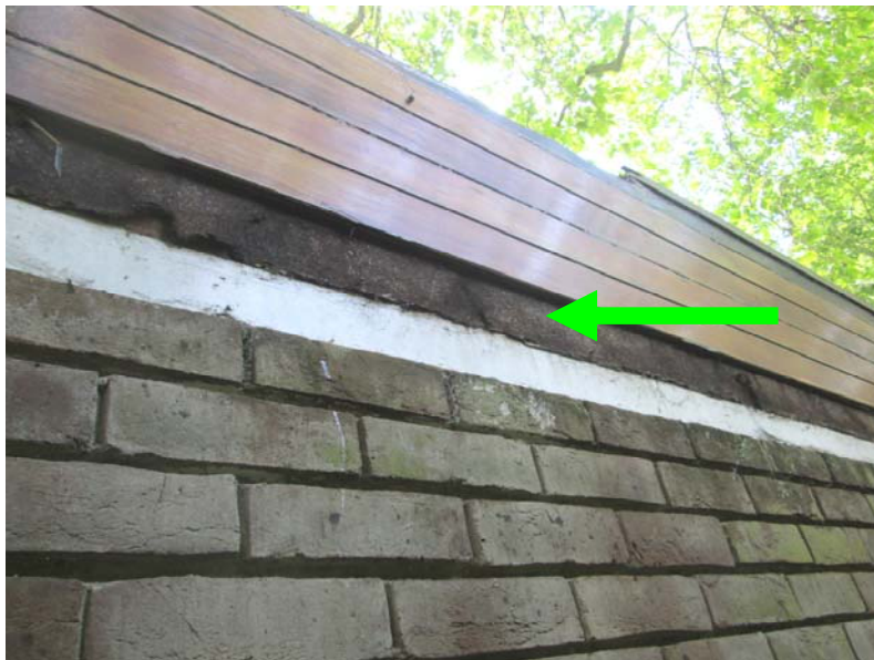
Sample 06 – Felt to upper side wall – external – no asbestos detected.
