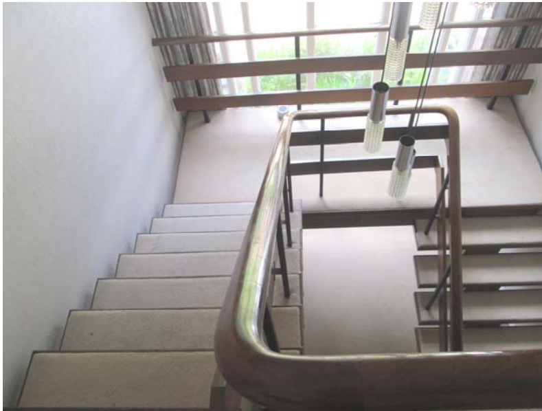
View of staircase, no asbestos detected.
