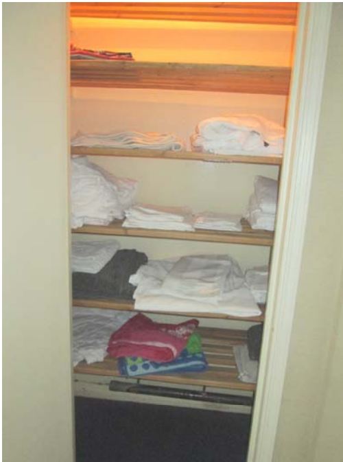
View of store cupboard, no asbestos detected.
