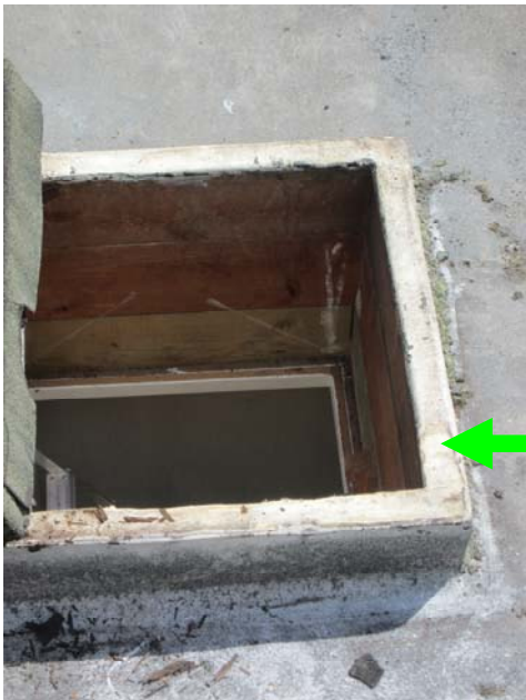
Sample 02 – Bitumen to loft hatch – flat roof - no asbestos detected.
