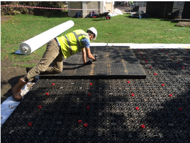
Installing Arbor Raft Two Units High
