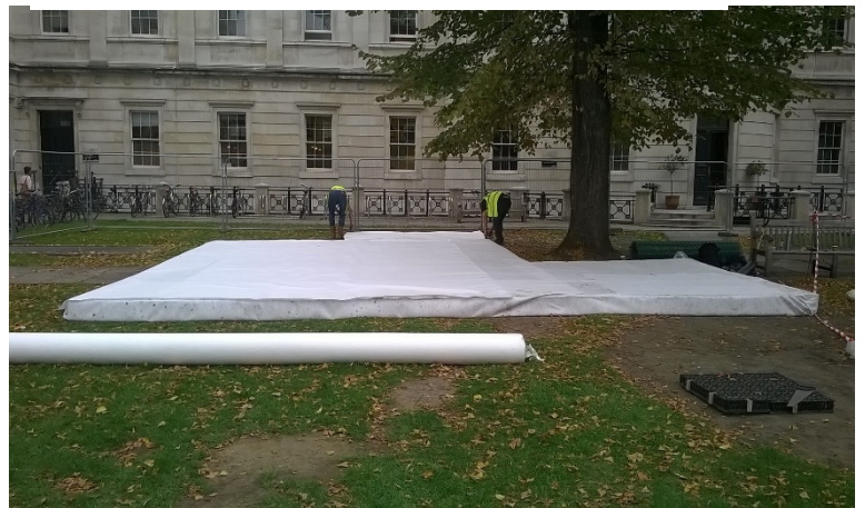
Section Of Arbor Raft Complete With Geotextile
