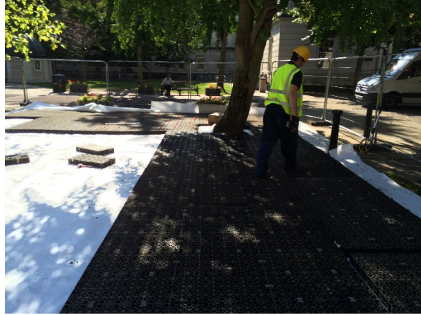
Section Of Arbor Raft Complete With Geotextile
