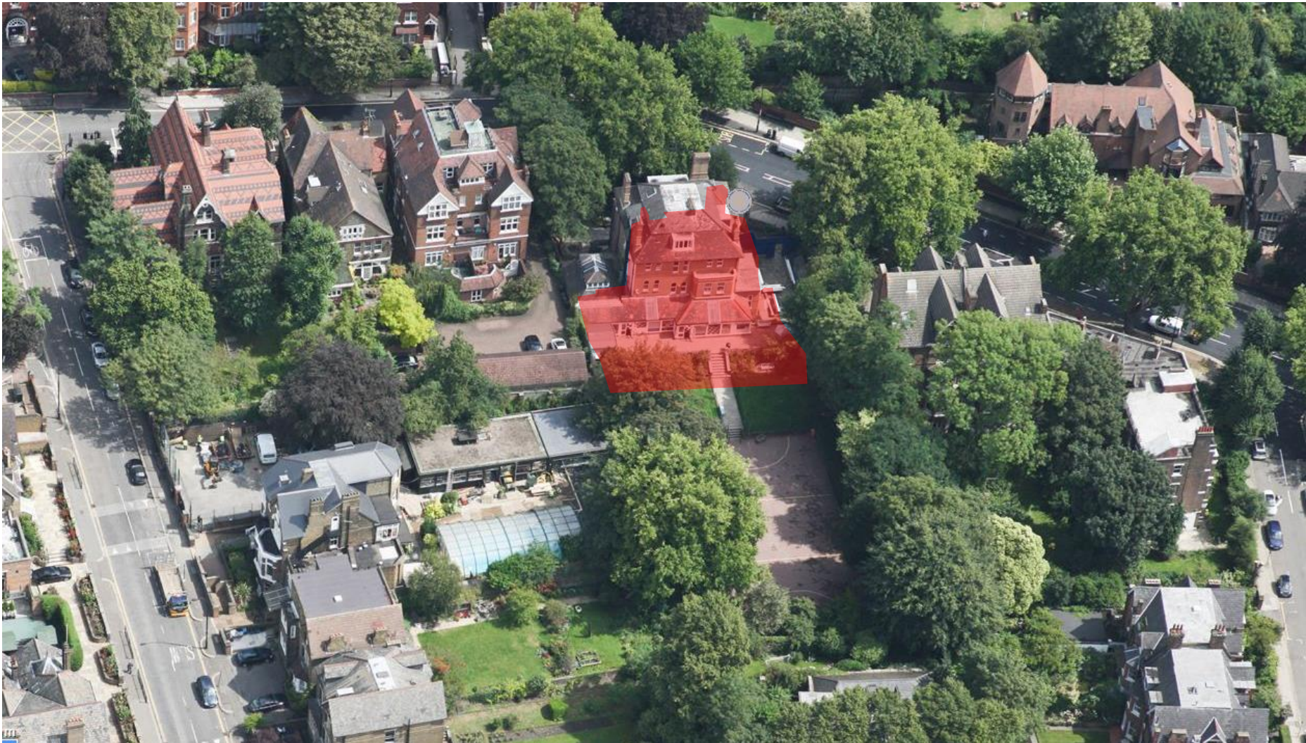
FIGURE 04 – BIRD EYE VIEW OF THE SITE AS EXISTING LOOKING NORTH
