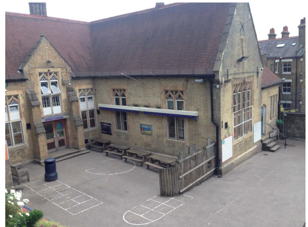
Fig 1 – Photograph of existing school building
