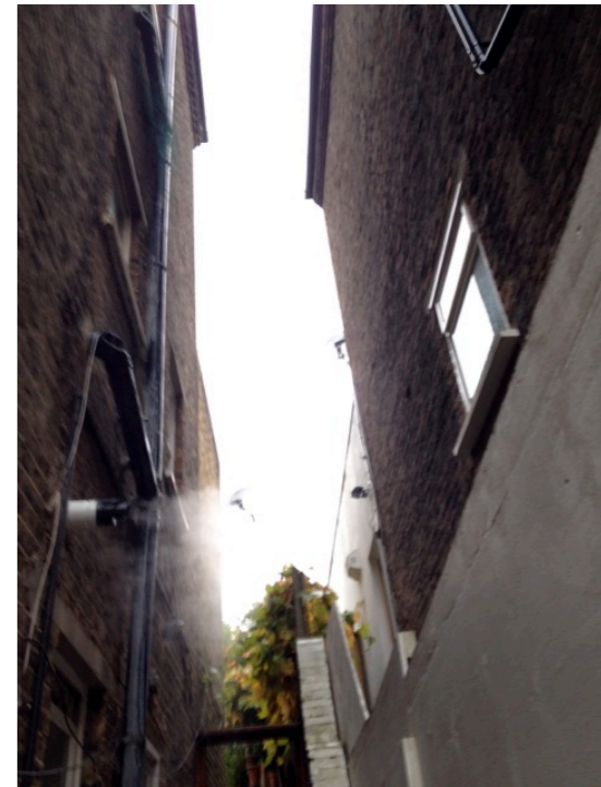
Side wall of no.15 & no.17
