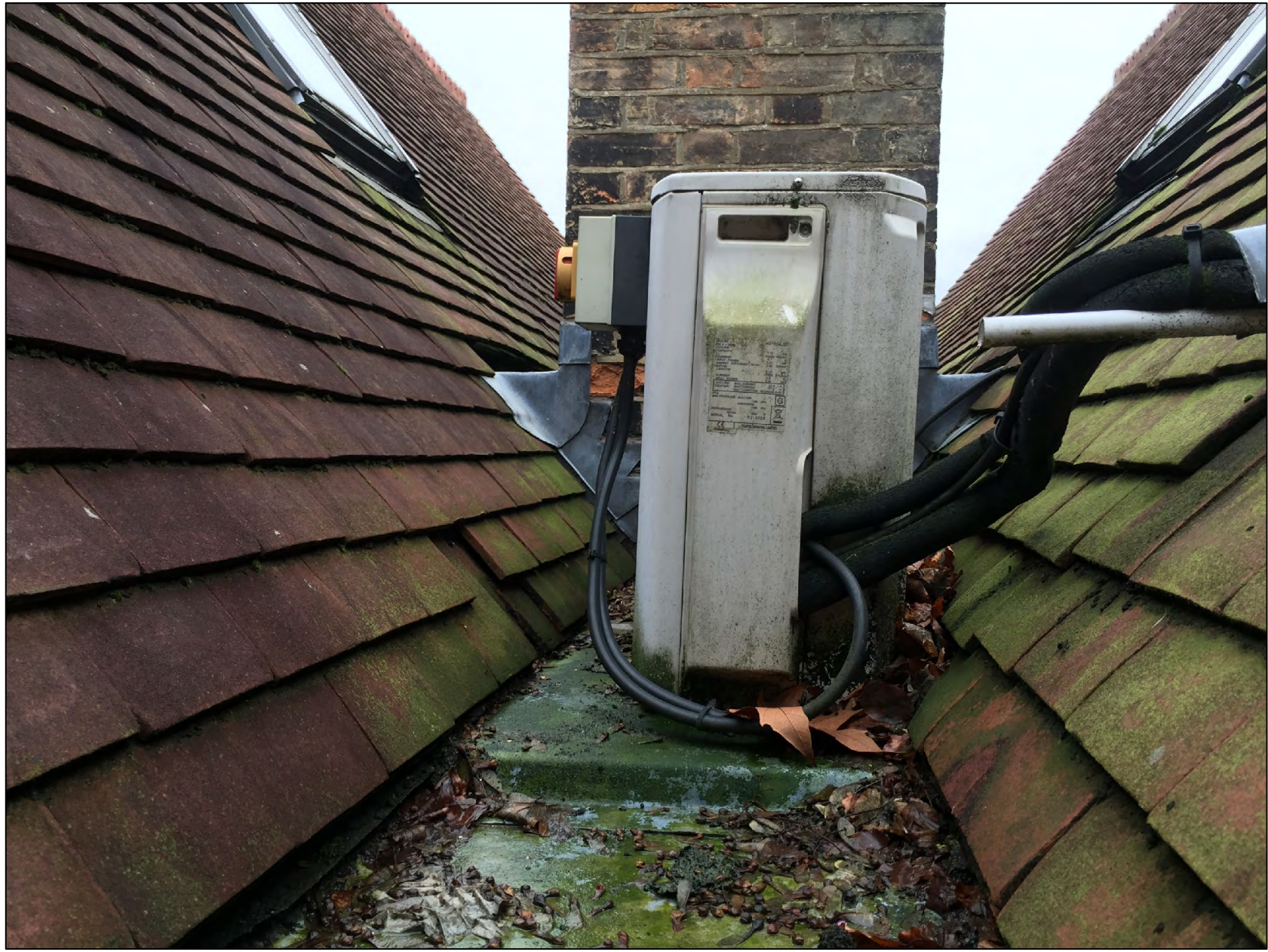
PHOTO A EXISTING ROOF MOUNTED EXTERNAL CONDENSER
