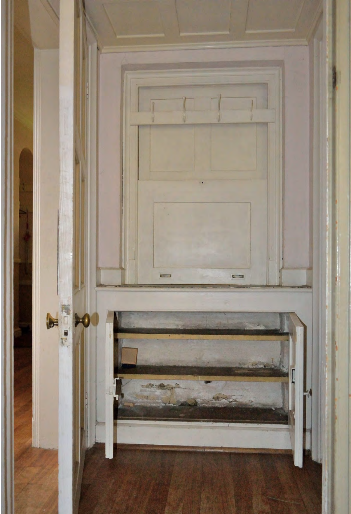
Fig 35, The kitchen / pantry lobby showing the closed serving hatch above a cupboard unit, which appears to be a historic detail. The wall behind also appears not to have been disturbed, and the skirting runs through.
