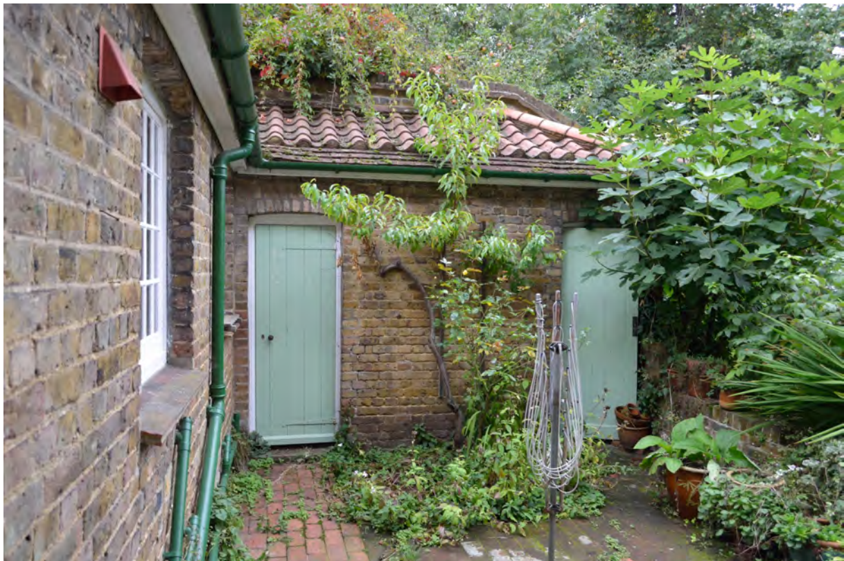
Fig 10. The end of the service range containing fuel stores within the small brick lined yard. The rounded tile hips to the roof are modern. .
