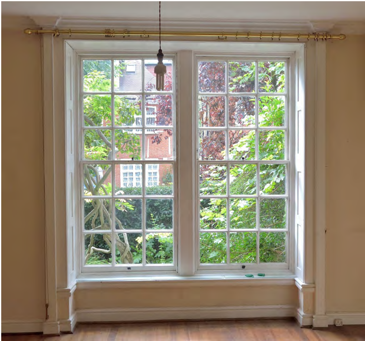
Fig 18, The original deep double sash window surviving in the dining room, with projecting architraves with pronounced moulded capitals and bases.
