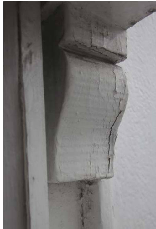
An example of one of the horns on the upper sash, which are in the Victorian style and show signs of having been machine worked.
