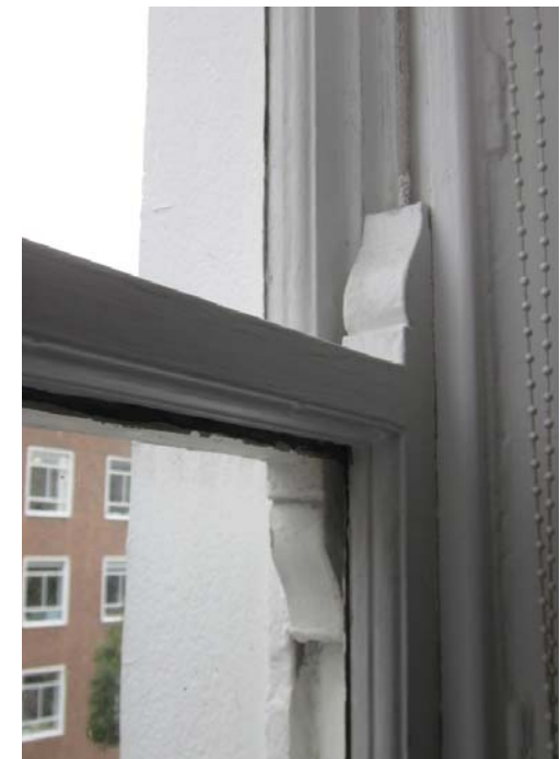
Detail of second floor front window showing the thick mid-rail with horns on both the upper and lower sliding sashes fillet and ovolo glazing bars in the Victorian-style.
