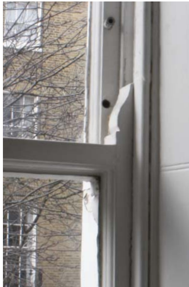
An example of one of the horned, wide mid-rails, which differ greatly from the original windows on the ground floor (shown on page 4).
