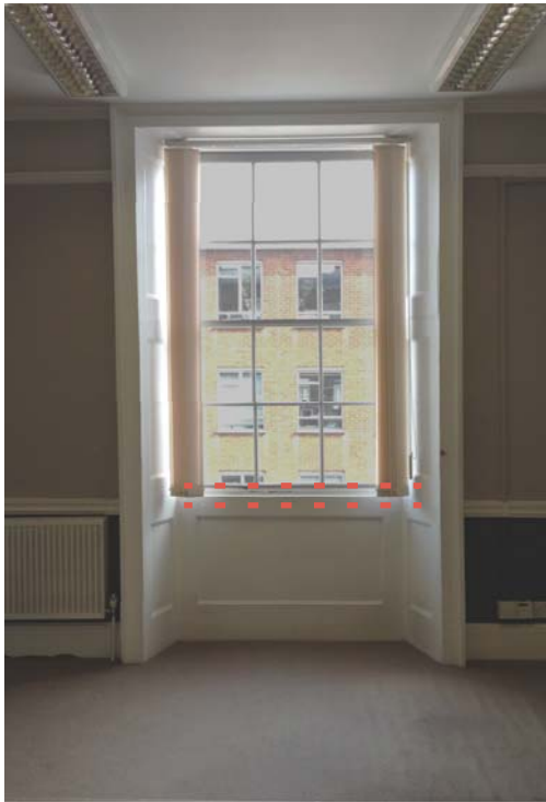
Second floor rear sash window viewed from interior highlighting the rot on the bottom rail.
