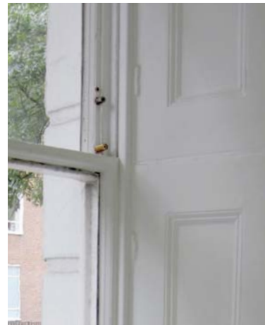
Original glazing bar without horns composes a refined and elegant window and is exemplary of the craftsmanship and quality of timber in the original sliding sashes.
