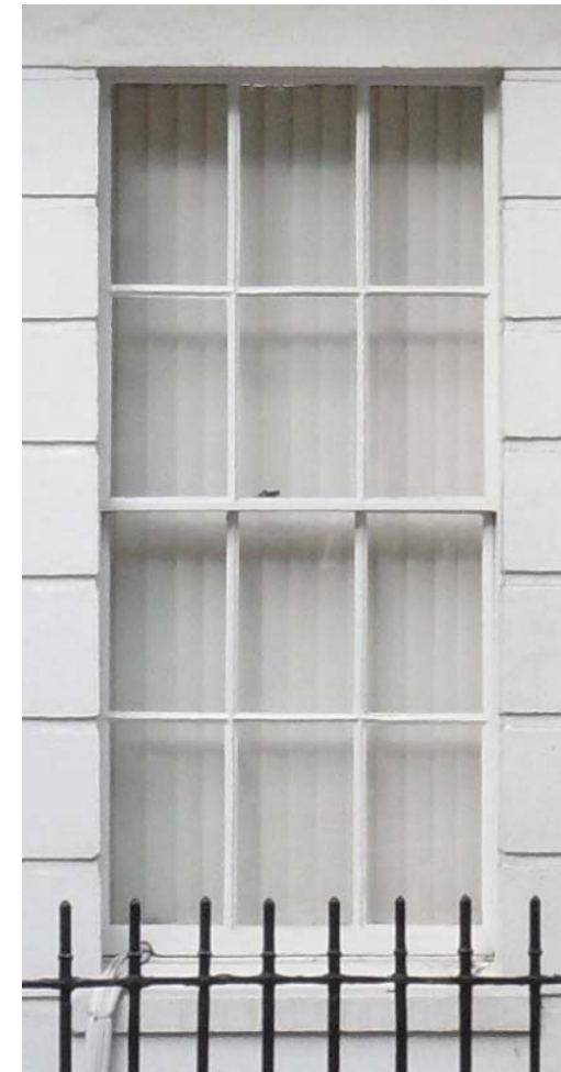
The fine glazing bars and mid-rail appear visually the same, with only a few millimetres difference in their width.
