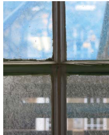
The profile of the 18mm broken lambs tongue glazing bars catches the light so as to accentuate their verticality and slenderness.
