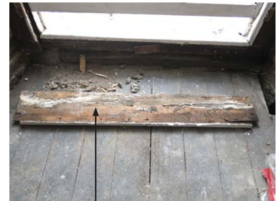
Severe damage to the skirting due to moisture ingress through the sill.
