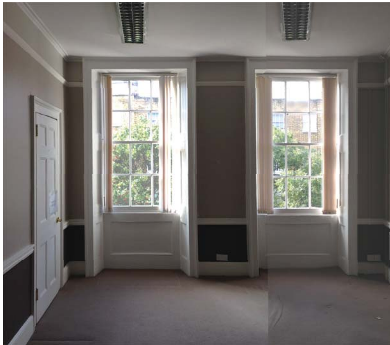
First floor front windows viewed from interior showing wide glazing bars and mid-rails that are much less fine visually than the Georgian originals.
