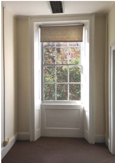
First floor front windows viewed from interior showing wide glazing bars and mid-rails that are much less fine visually than the Georgian originals.
