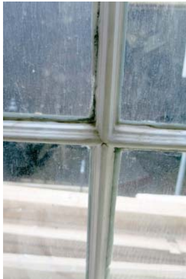
Close up of 18mm 'broken lambs tongue' glazing bar, whose delicate profile reflects the light, emphasising the verticality and slenderness of the window.
