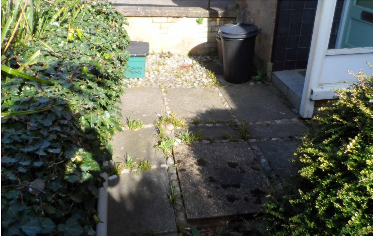
Photo 5: Concrete manhole cover within the front garden, indicating the possible position of a lateral sewer. Note gully in pebbled area near boundary.
