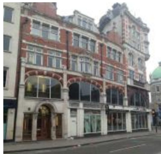
01 Existing Building P01
