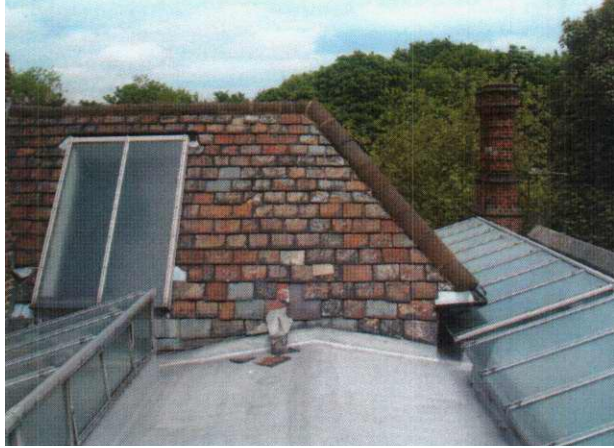
Figure 1.0: Existing Rooflights above The Studio
