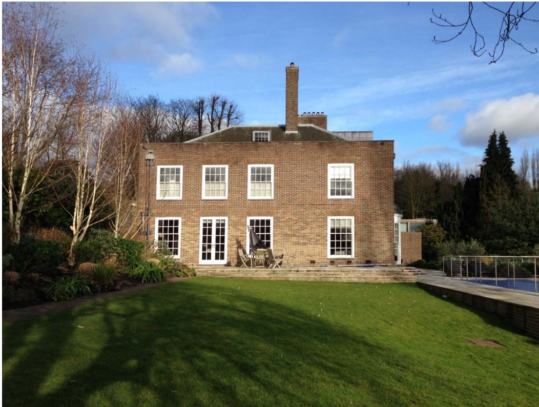
Figure 3 – Proposed Side Elevation – The proposed dormer is in line with the windows on the lower floors. The new dormer is designed in a traditional manner, and it matches the style of the existing house
