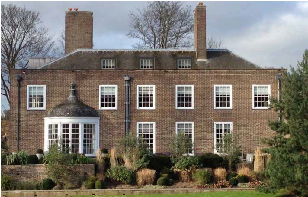
Figure 2 – Proposed Rear Elevation showing new dormers in line with the windows below The dormer windows are designed to match the style of the existing house
