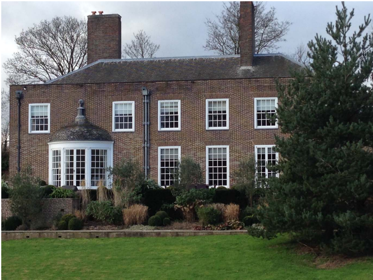
Figure 1 – 10 Fitzroy Park, view of rear elevation as existing
