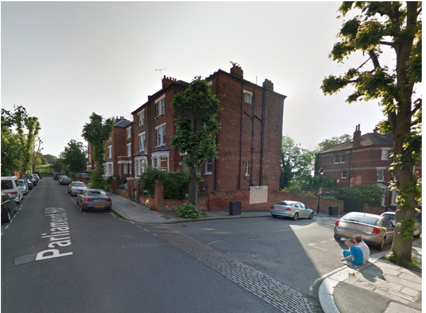
Side elevation view from the street
