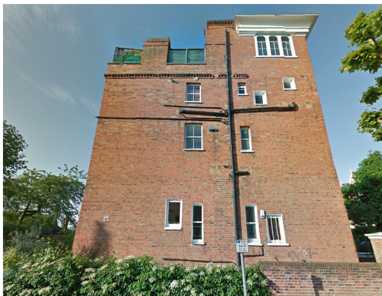
Windows to side elevation of house opposite at 60 Parliament Hill
