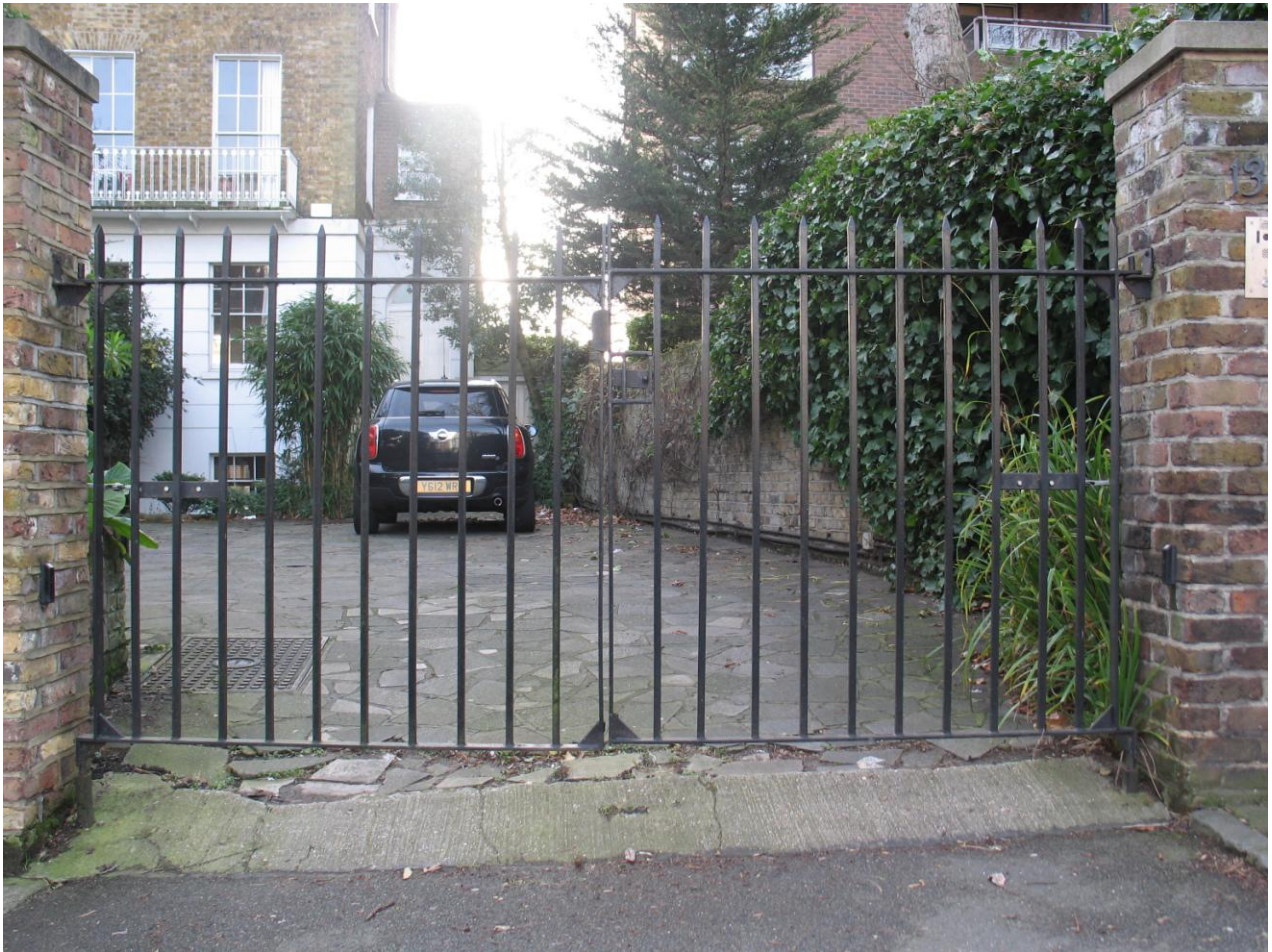
Front main gates at 133 Haverstock Hill – Simply in design no central folding with pointed top finish, in a metal finish
