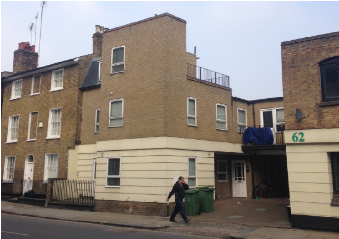
Above: Subject site and surrounding development, including 64 (Listed Building, left), 62A (centre) and 62 Highgate Road (right).
