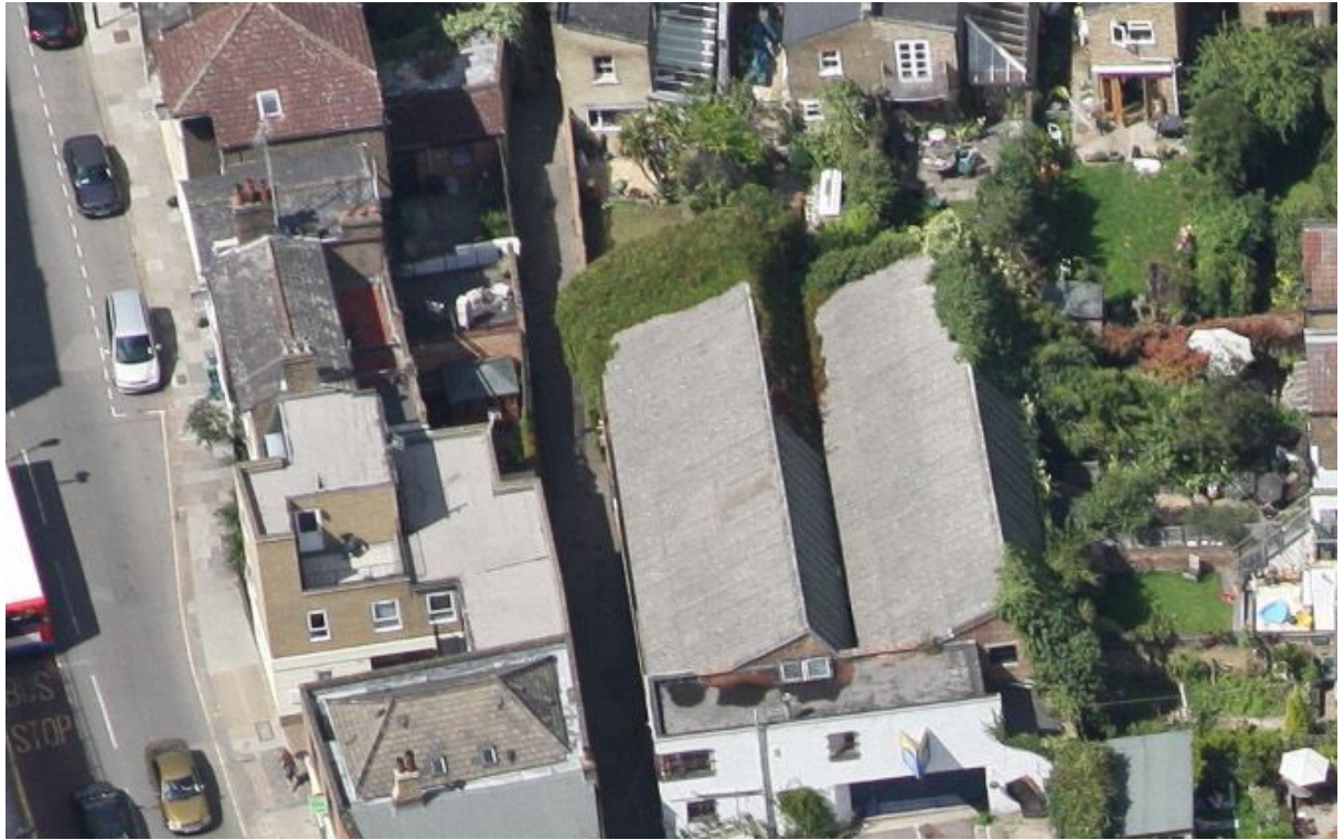
Above: Aerial Photograph looking north over subject site (source: www.bing.com )
