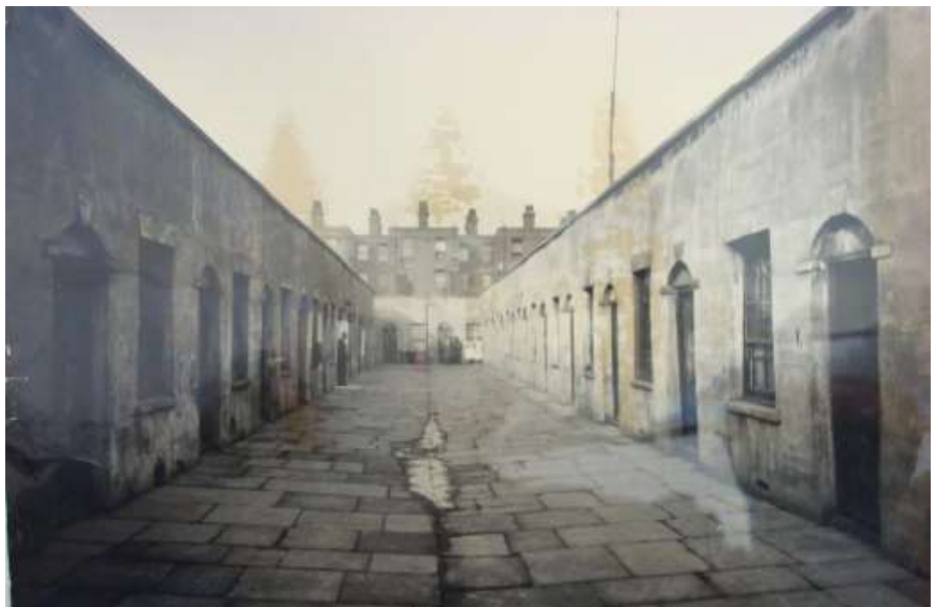
Figure 7: Equity Buildings, Looking North, 1928
