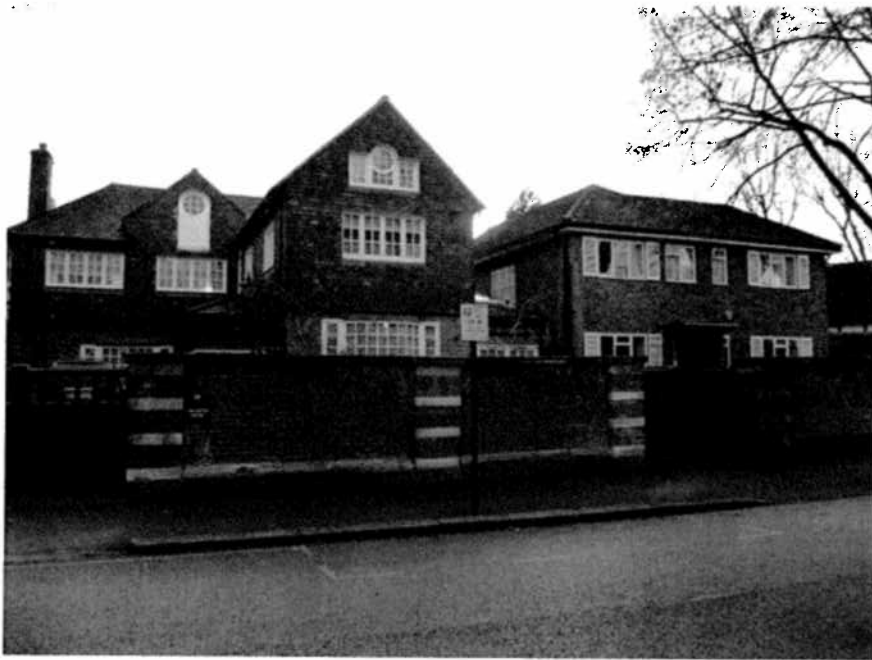
Fig. 3 Nos. 24 and 26 Lancaster Grove
