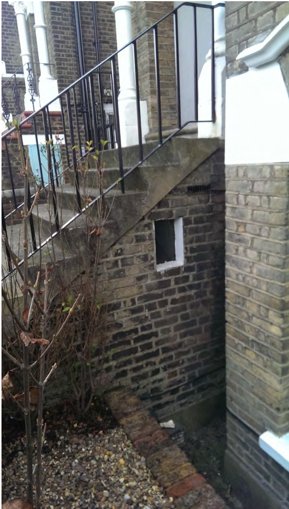
Front View – Side under staircase
