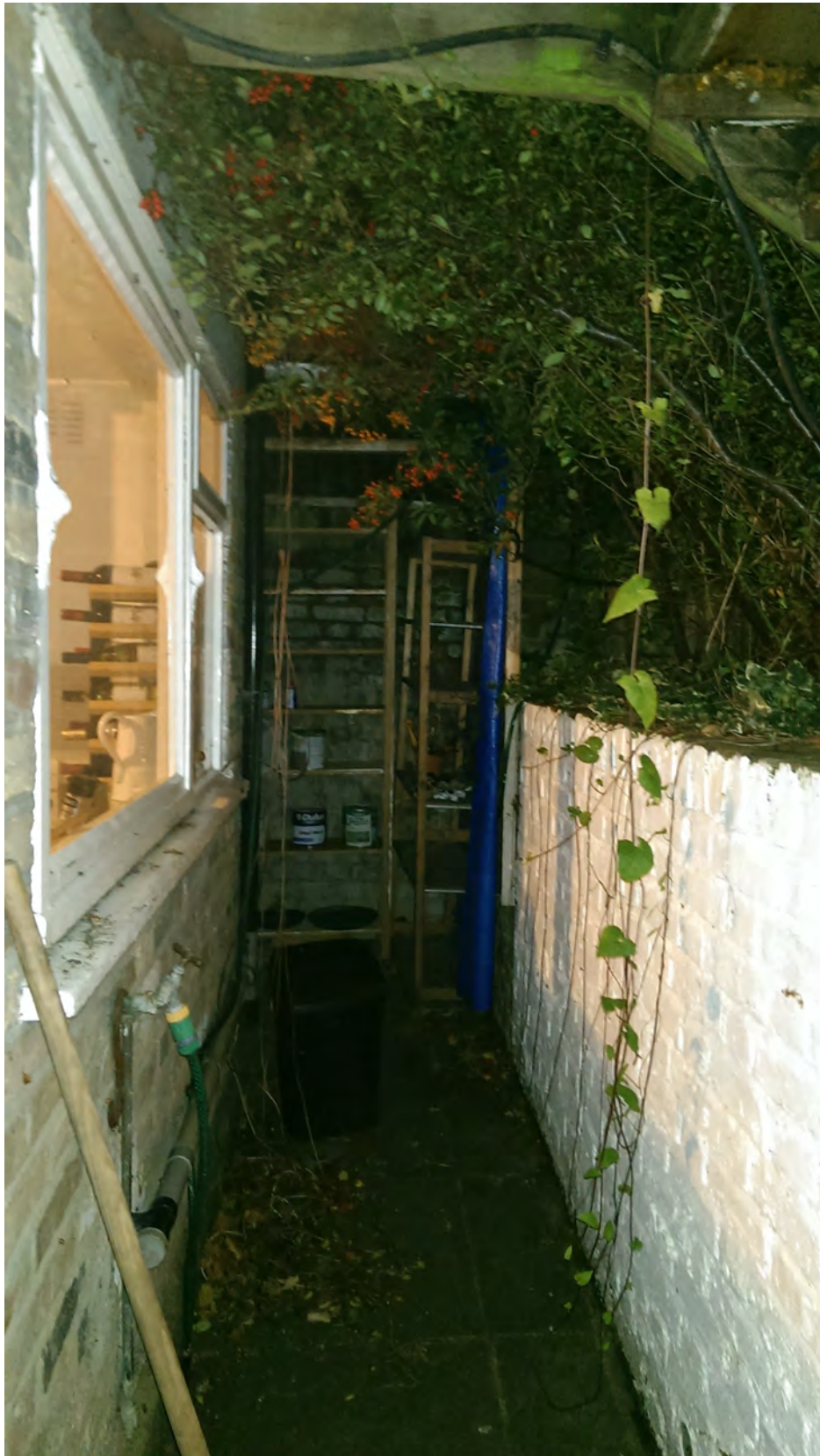
Rear View - Kitchen Window.
