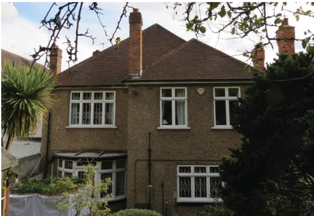
fig 4. Rear elevation photograph of the existing house
