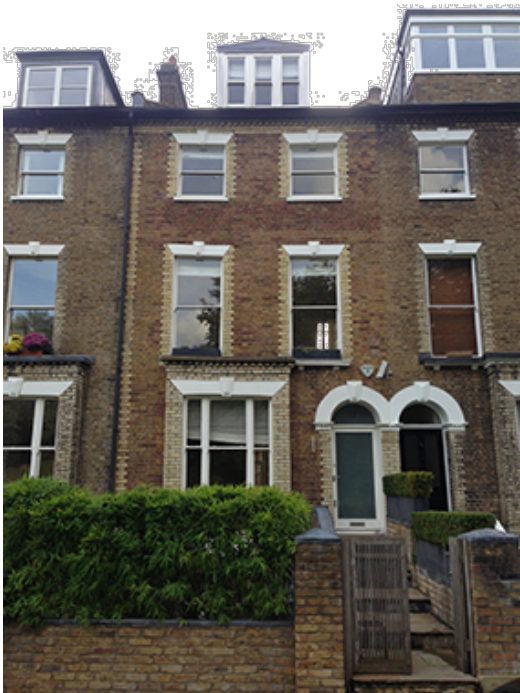
3 Christchurch Hill Front Elevation showing existing dormer
