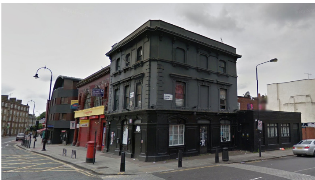
Figure 1: Image of existing building
