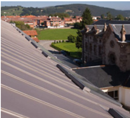
Zinc standing seam roof detail examples
