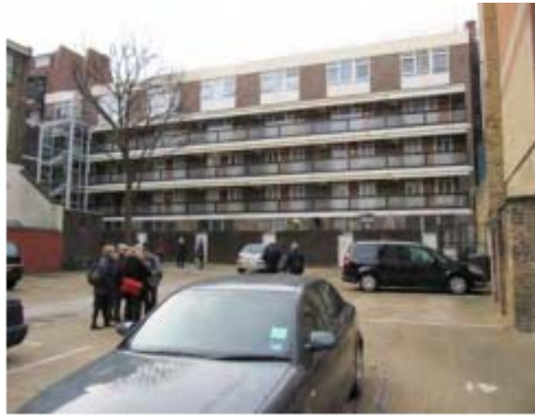
2- The existing space to the rear of Devonshire Court is dominated by car parking areas at present.
