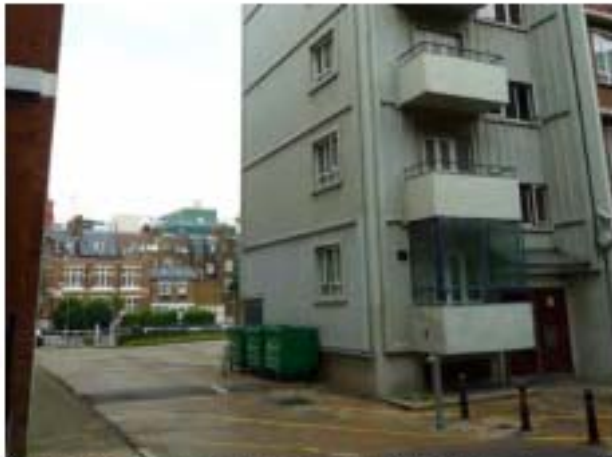
3- View of the south end of Blemundsbury with cramped main entrance to right and bins overflowing outside building due to lack of ground floor storage area.
