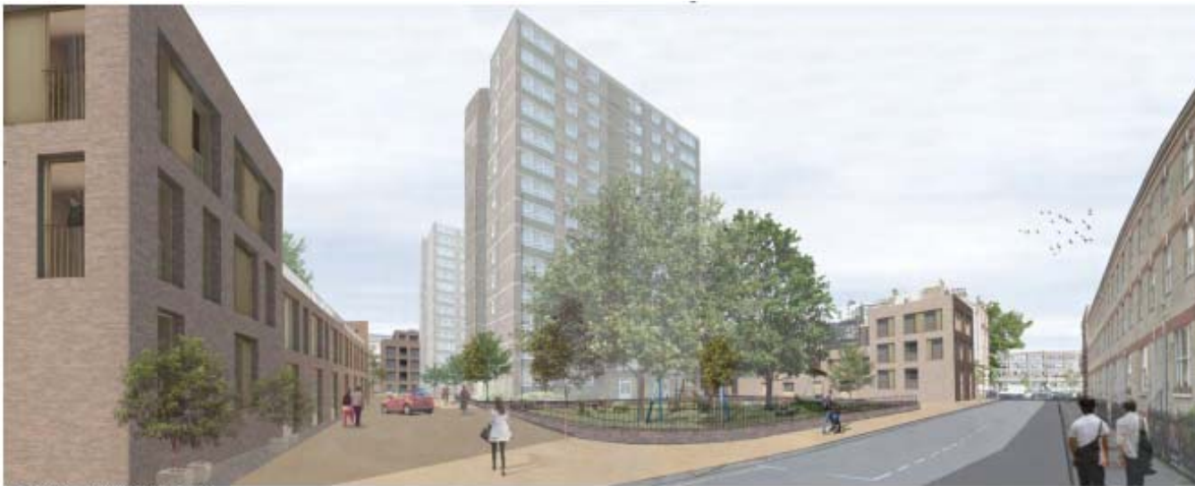
View looking west from Orde Hall Street
