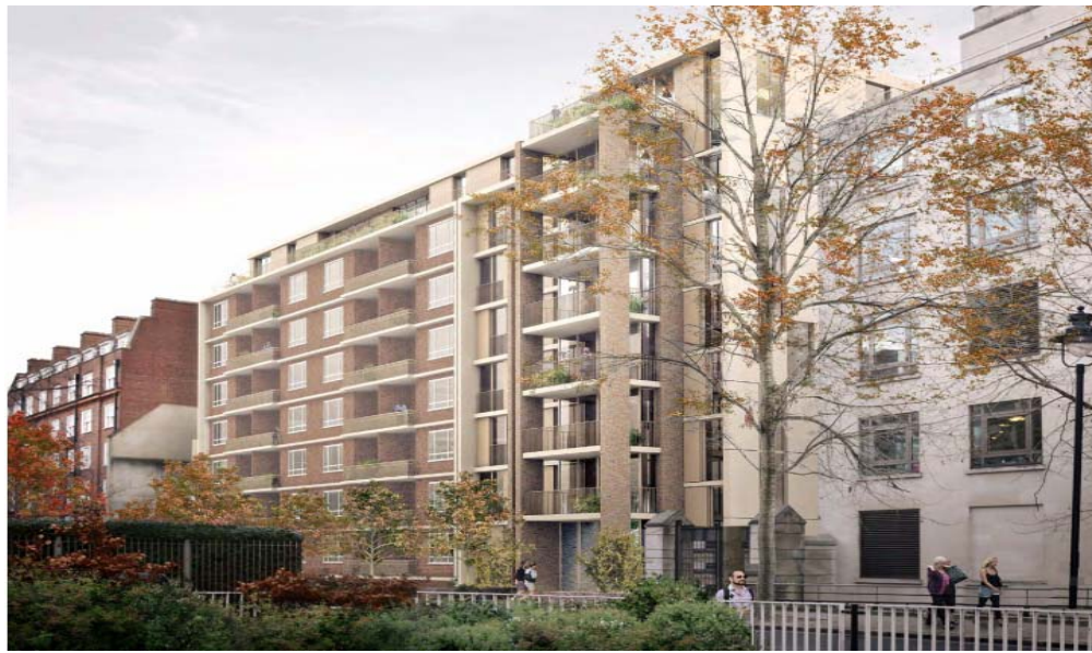
Overbuild and side extension
