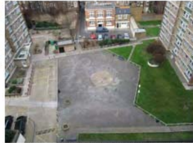
4- The main open area between the two towers. This space is currently dominated by poor quality hard-surfacing and underused grass areas.
