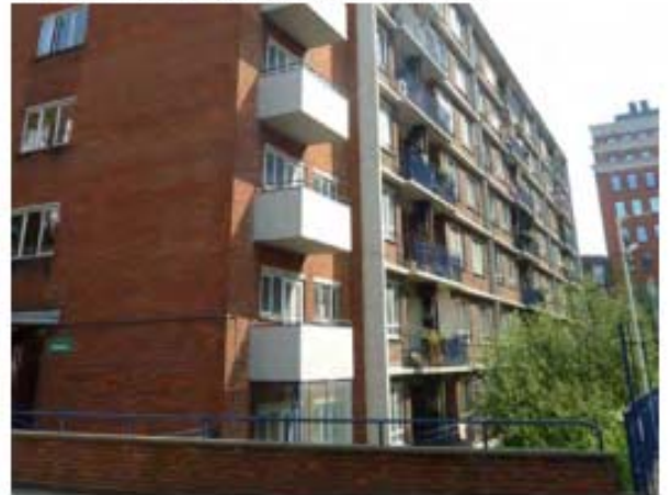
6- View from New North Street showing existing unused washroom balconies.
