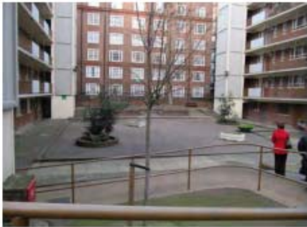
1- Existing courtyard viewed from south
