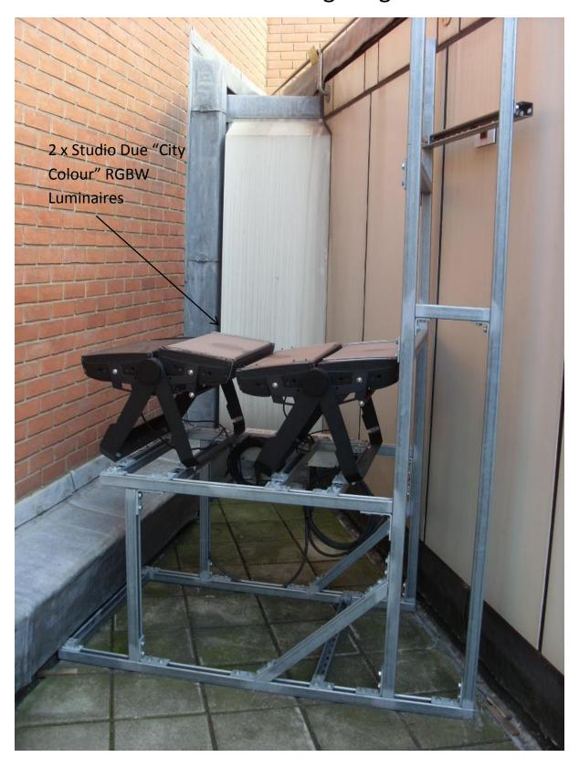
Studio Due City Colour Luminaires mounted on Uni Strut framework at the base of the Clock Tower
