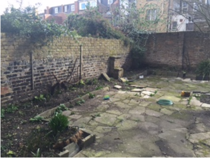
Existing garden wall between no.5 and No.6 Gloucester Crescent.
