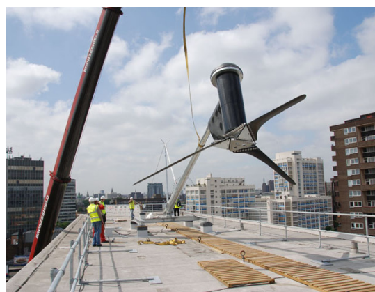
A building-mounted 6kW Proven wind turbine
