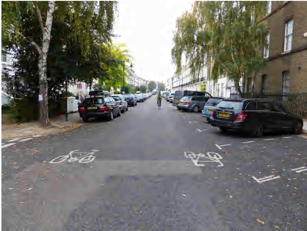
Figure 3 Existing Road Condition along Gloucester Avenue – North-westbound
