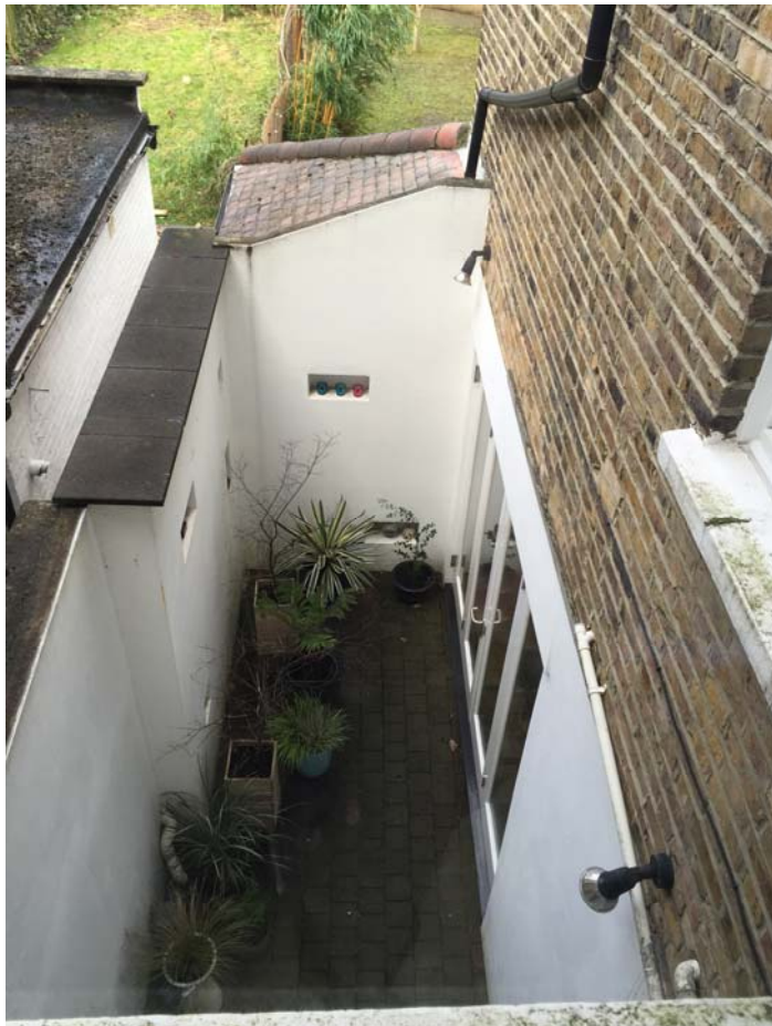
Existing lightwell adjacent to original closet wing
