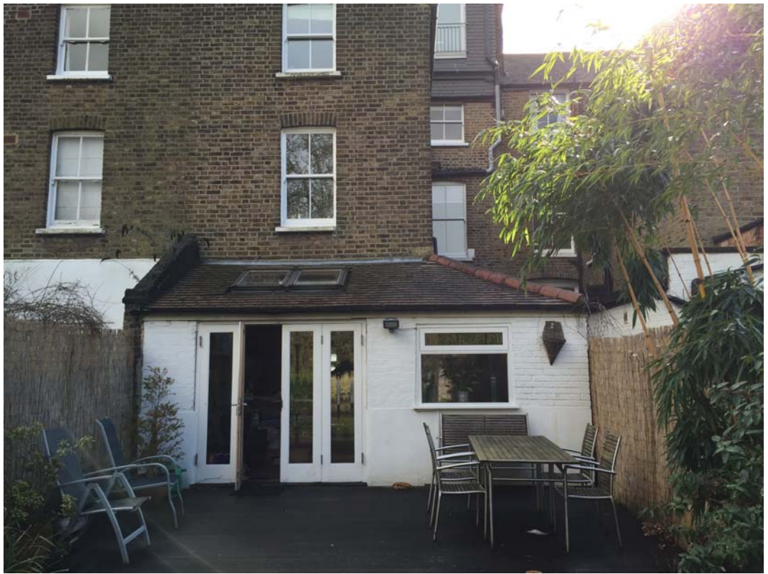
View to rear existing extension
