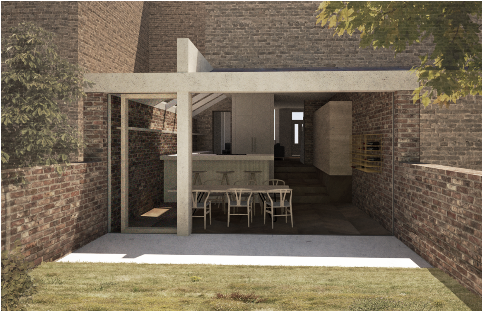
Visual 1: showing the proposed rear extension & highlighting the connection of the interior and outdoor space. The extension is designed & materialised to display juxtaposition between a brick dominated surrounding and new, precast concrete structural elements (lintel & main beam) along with double glazed panels. Our careful choice & differentiation of materials supports & retains a visual footprint of the original rear extension and helps the new structures to distinguish themselves.
