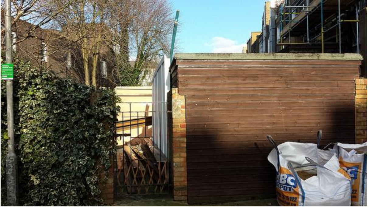
Shed to be demolished – from Kingstown Street
