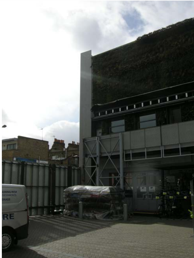
Fig 12 The area of proposed development in the courtyard, looking south-west (MOLA photo, taken 23/02/14)
