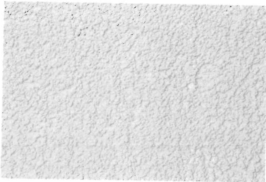
Render: West,elevation Rockwool topcoat - 1.5mm aggregate - Colour ref 8C46
