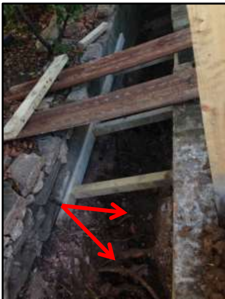
Image 1: Root investigations along the retaining wall revealed a number of significant roots
