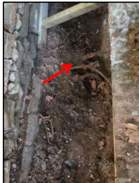
Image 2: The roots found beneath the retaining wall need to be severed to accommodate piling works
