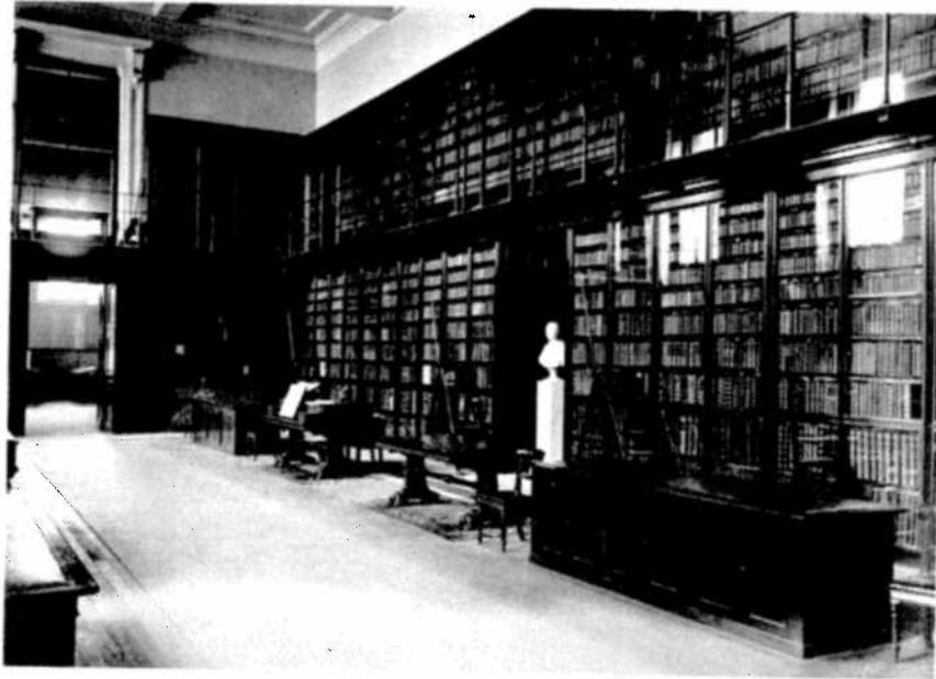
Original arrangement (from Grenville Library side)
