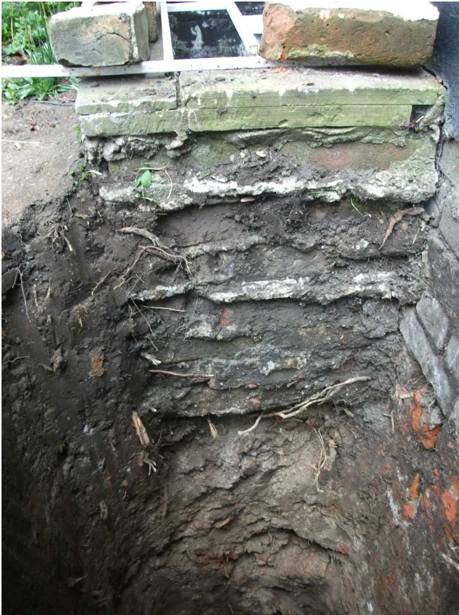
Plate 3: Looking at the footing of the lightwell in TP1.
