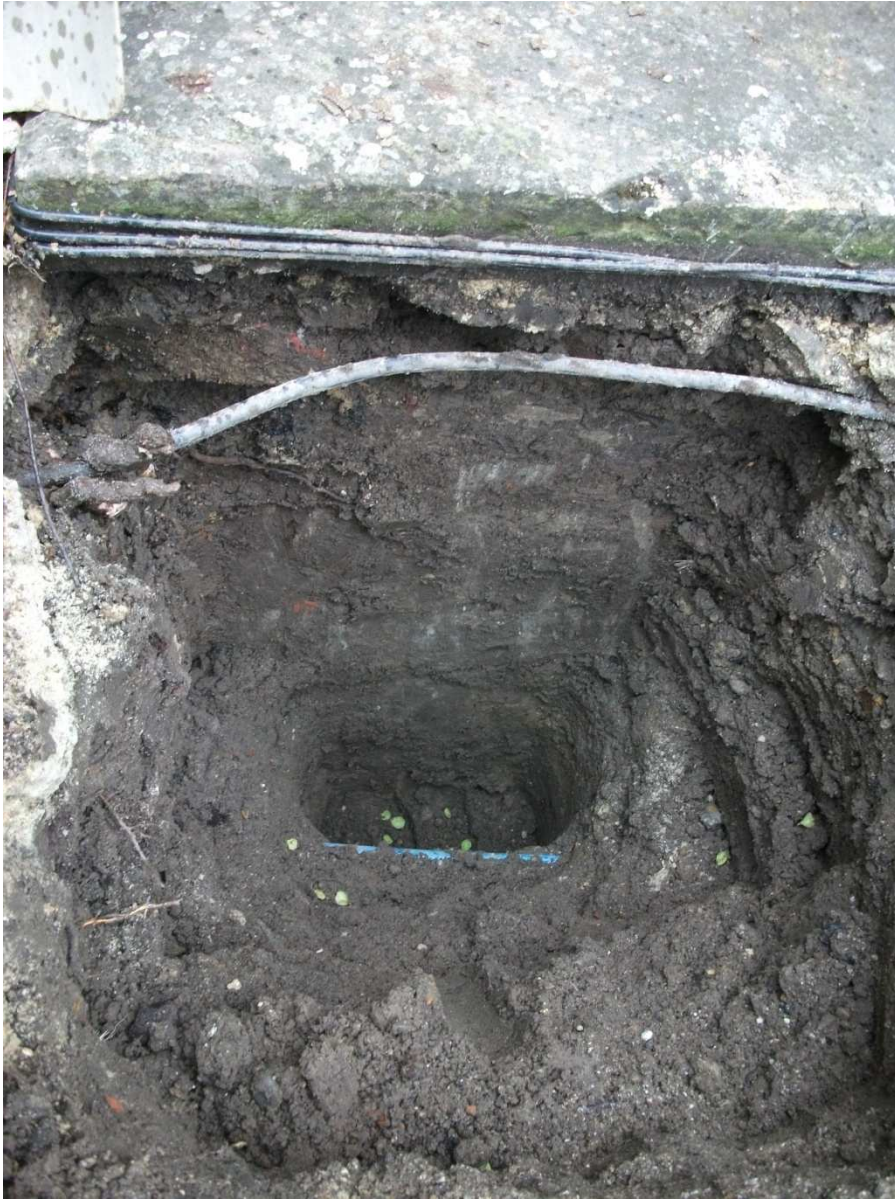
Plate 5: Looking at wall of covered lightwell in TP2.
