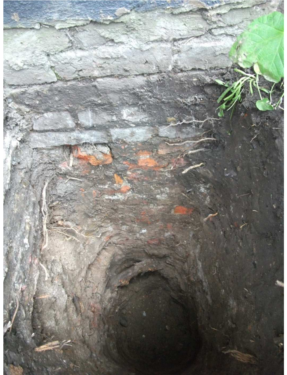
Plate 2: Looking at the basement wall in TP1.
