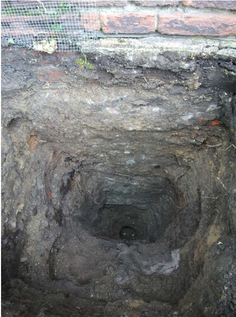
Plate 7: Looking at basement wall in TP3.
