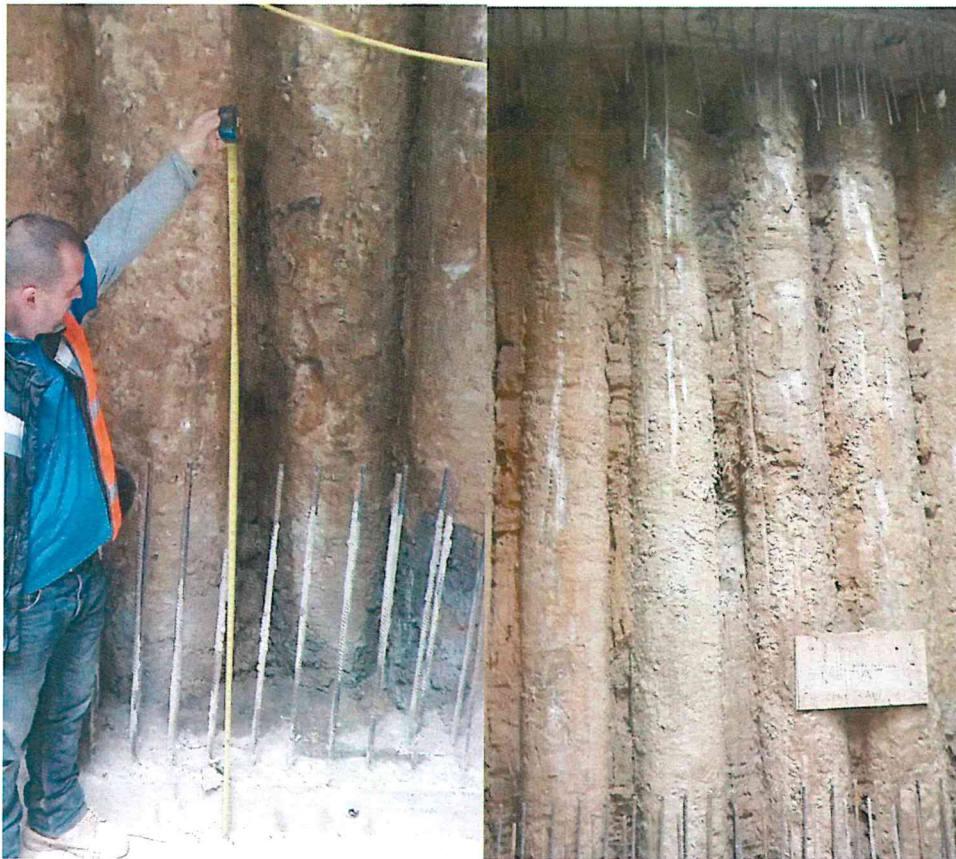
Photographs of Basement Construction at 4 Upper Terrace 29.09.2014 indicating contiguous bored piling and minor water seepage at 126.5m AOD
