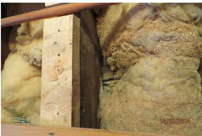
P11 – Third floor original joists and modern firring pieces.
