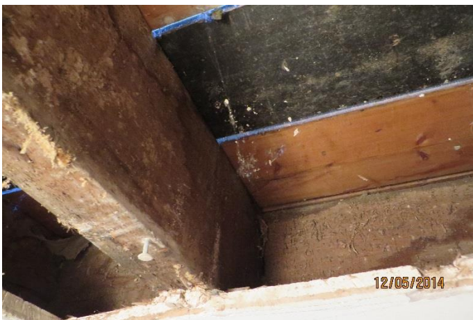
P3 – Underside of ground floor in rear hall.
