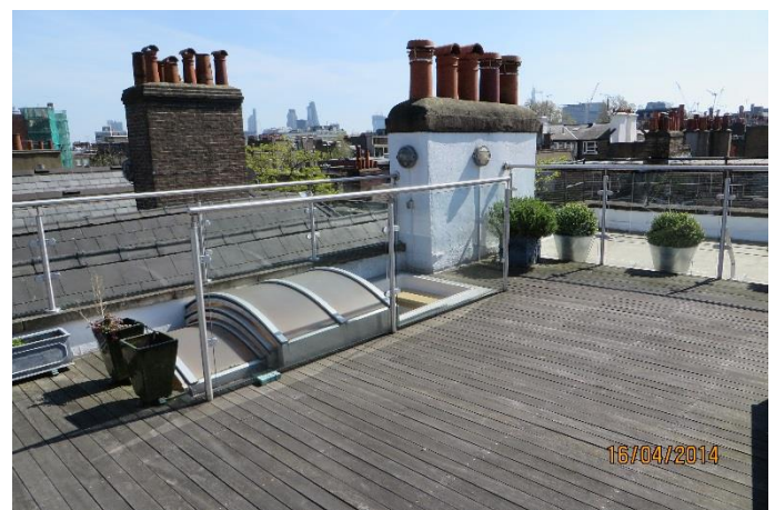
P12 – Sliding roof hatch.
