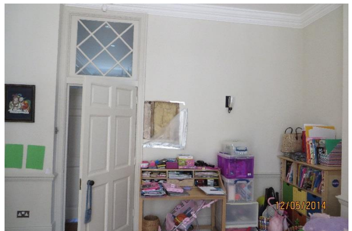
P6 – G Floor existing single style door between front and back rooms.
