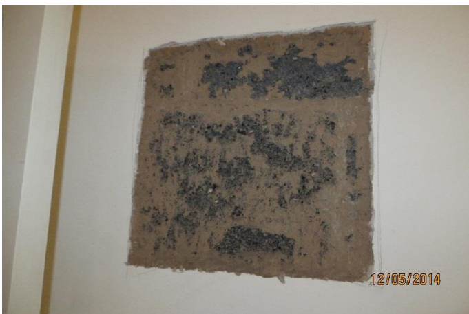
P5 – LG. Blockwork partition between front and back.
