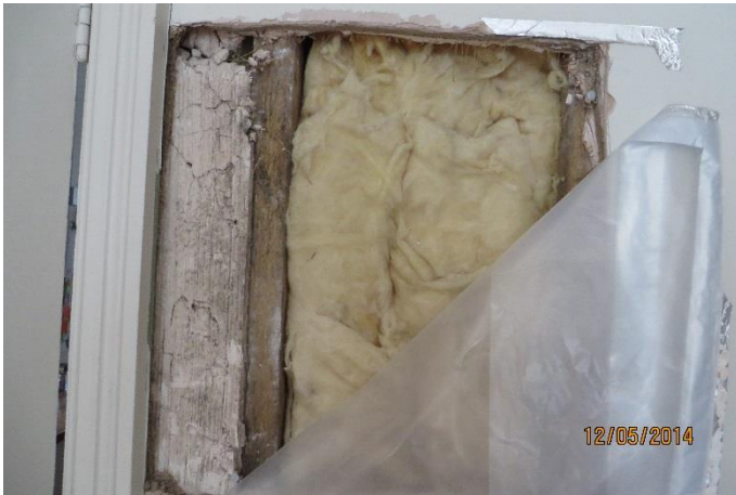
P7 – G Floor. Modern construction between front and back rooms.
