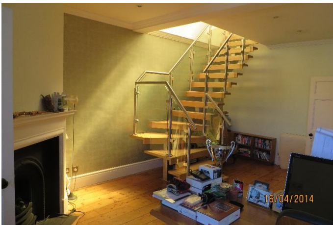
P9 – The floor existing steel framed staircase.
