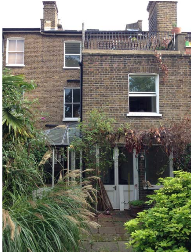
21 Boscastle Road - Existing rear elevation
