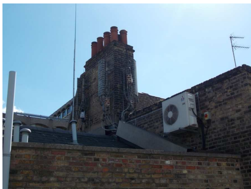
Fig. 1: Existing antennas mounted on support poles
