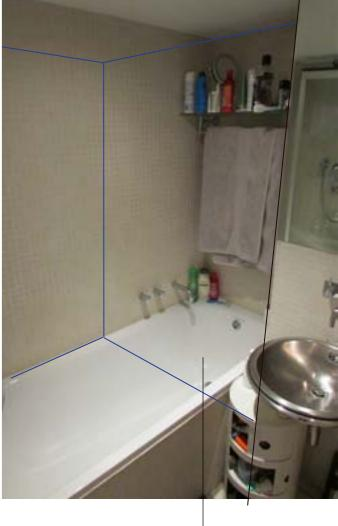
NON ORIGINAL WALL REMOVED AS PART OF BATHROOM ENLARGEMENT SIZE OF UPPER GROUND FLOOR BATHROOM EXTENDED INTO REAR BEDROOM.
