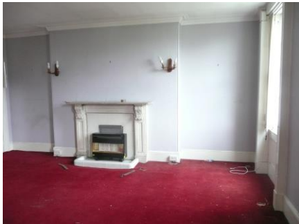
Fig 4 Existing Living Room to Flat Third Floor
