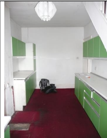
Fig 8 Existing Kitchen to Flat Third Floor
