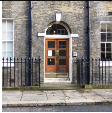
Fig 2 Main Entrance Door No4 Raymond Buildings
