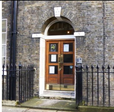
Fig1 Main Entrance Door No3 Raymond Buildings
