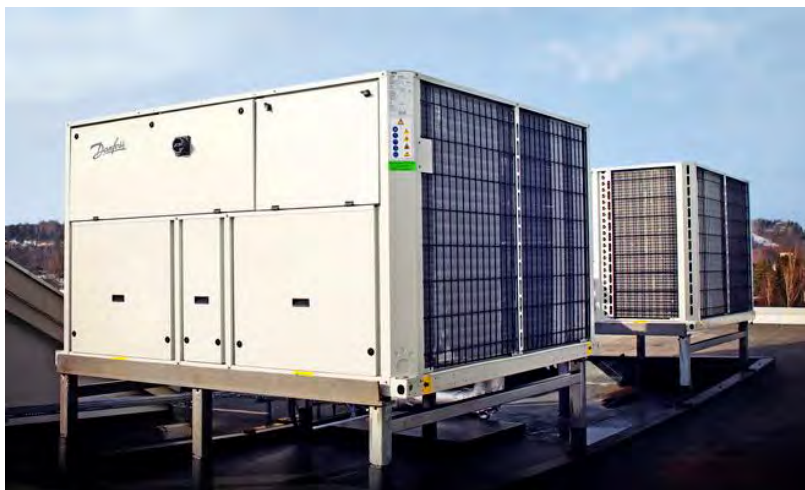
Figure 13: Typical commercial air source heat pump condenser units positioned on the roof of a building
